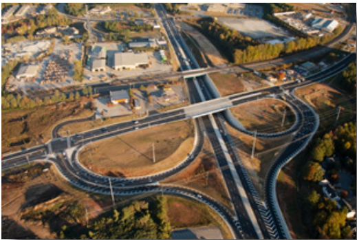
Figure 6: At-Grade Intersection to Grade-Separated Interchange
